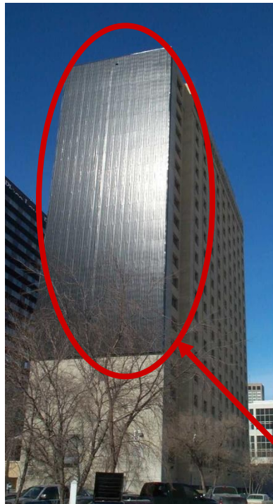
185 Smith Street, Winnipeg, Manitoba, Canada Photo source: Manitoba Housing Authority
